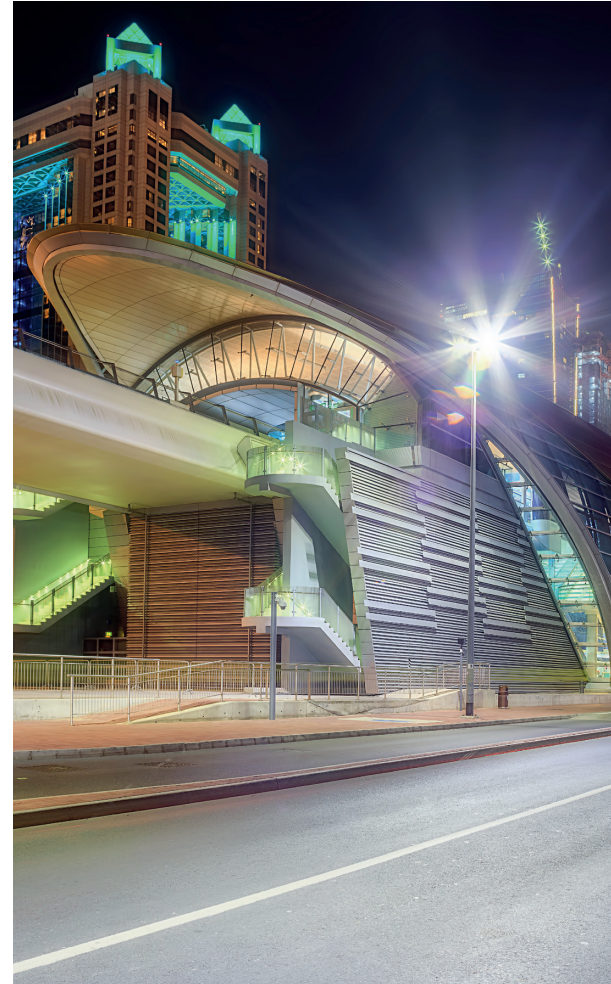
Dubai Burj Khalifa metro station – protected by SteelMaster
